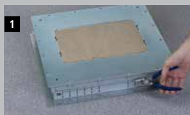
1 Trim the trunking entries
