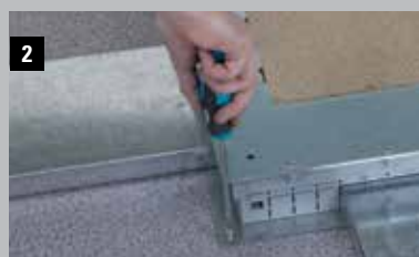
2 Insert the trunking and screw to the floor
