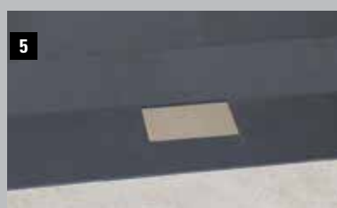
5 Fit the lining
